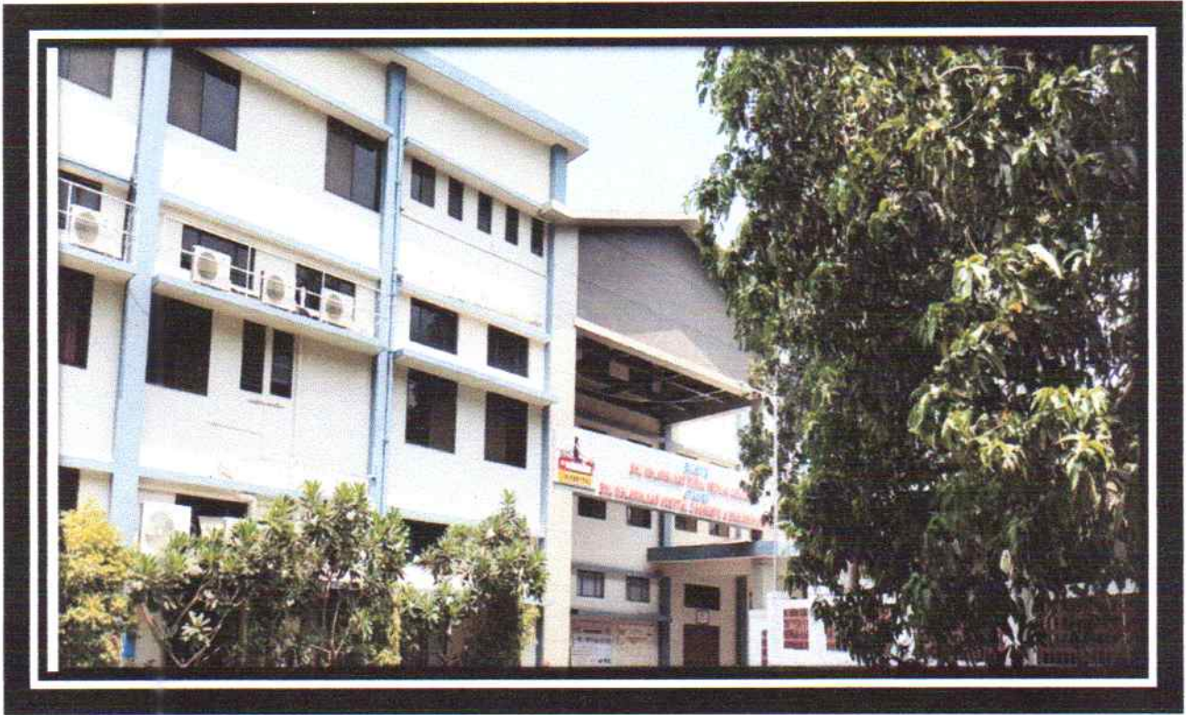
BKL Walawalkar Hospital Dervan
