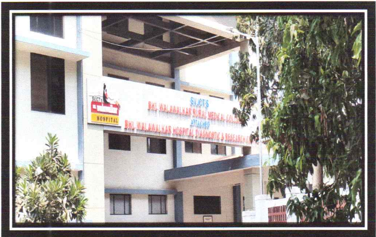
BKL Walawalkar Hospital Dervan
