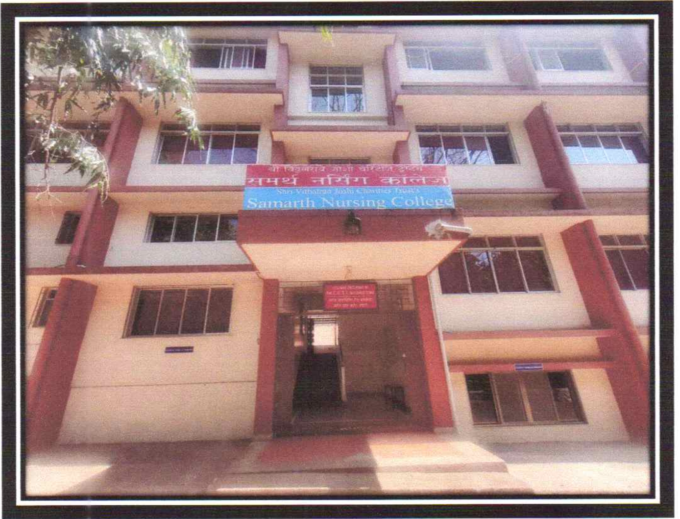
Samarth Nursing College Building
