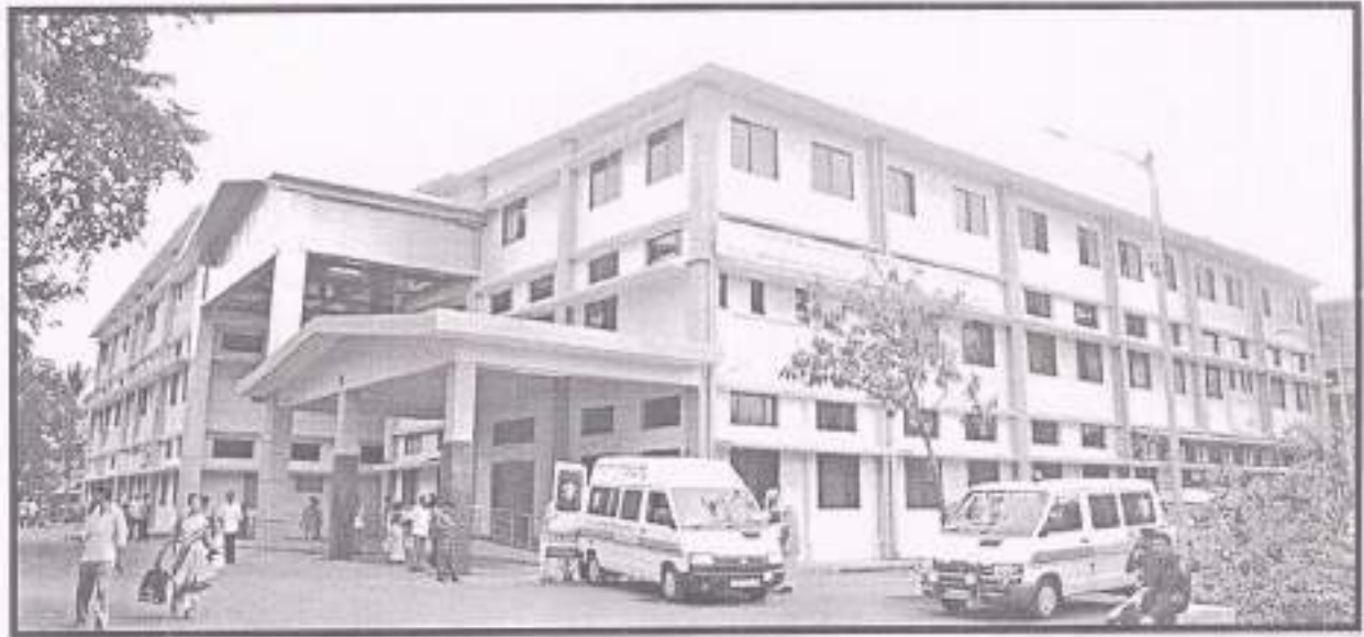
BKL Walawalkar Hospital Diagnostic & Research centre attached Rural Medical College ( IPD Building)
