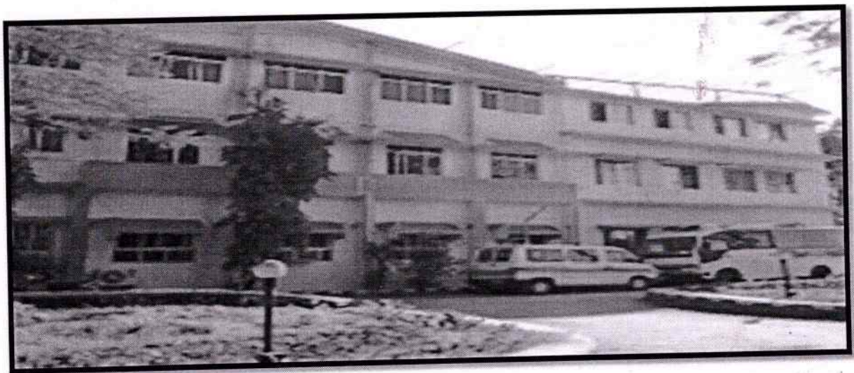
BKL Walawalkar Hospital Diagnostic & Research centre attached Rural Medical College ( OPD Building)
